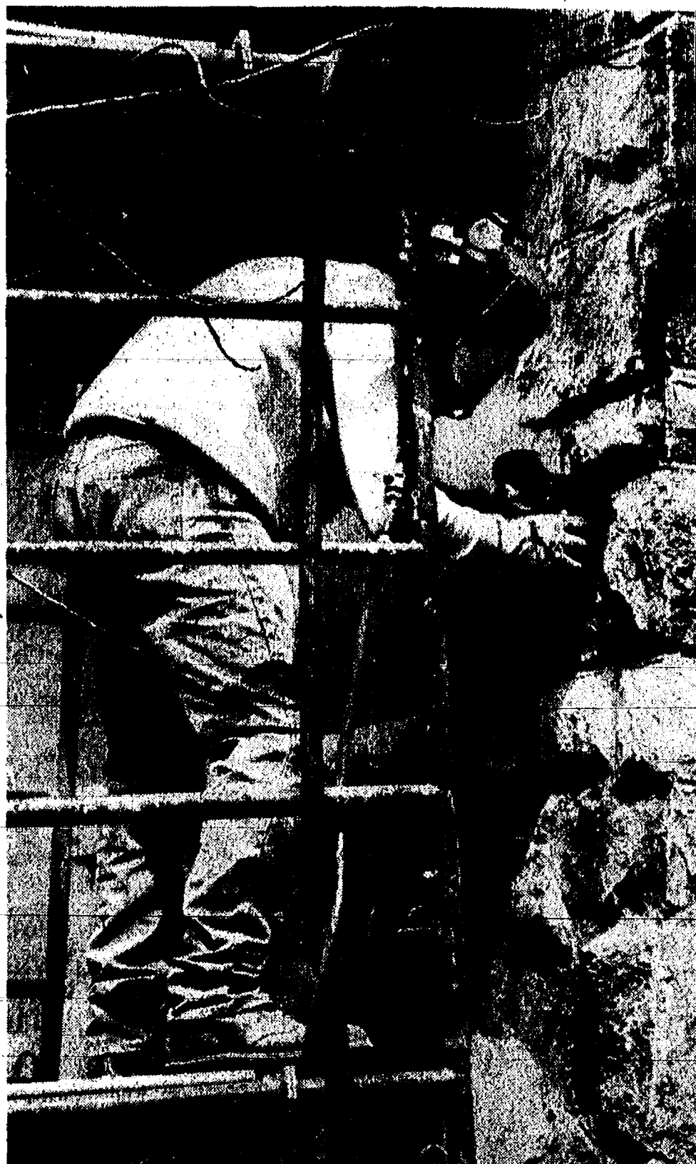
THE BEAUTIFUL STONEWORK of the Chelsea First United Methodist church on Park St. got a little tender loving care last week as workers restored the mortar joints between the stones, a process called tuck pointing.
